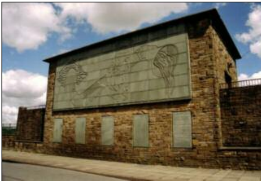
The artwork at Heaton Park Pumping Station. Photo: Creative Commons
